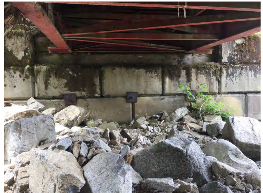
Left Bank Abutment when facing downstream
