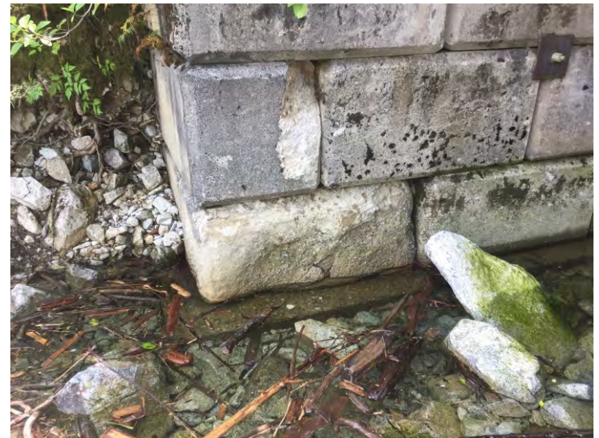
Bottom lock blocks at downstream right abutment
