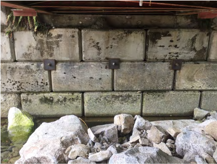
Right Bank Abutment when facing downstream
