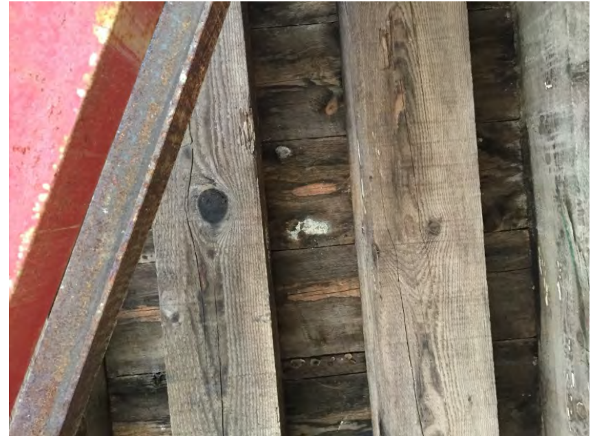
Deck from underneath
